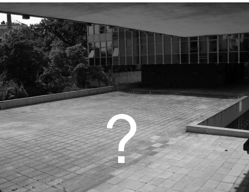
Flat roof of IPR Praha
