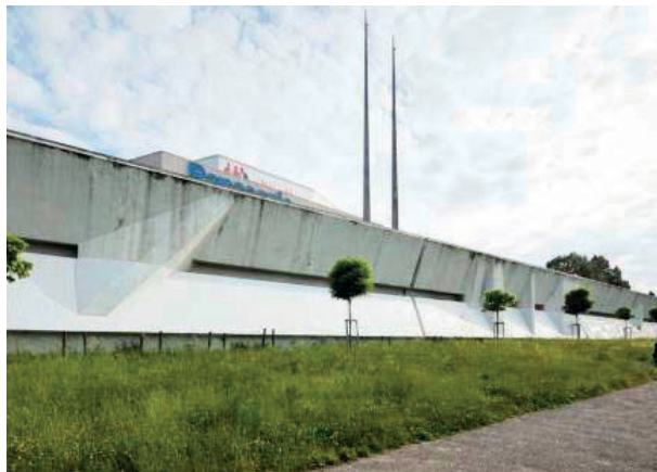
001 Supporting walls by the Nusle Bridge Stanislav Kolíbal (1968) [Prague 4, Vyšehrad]
